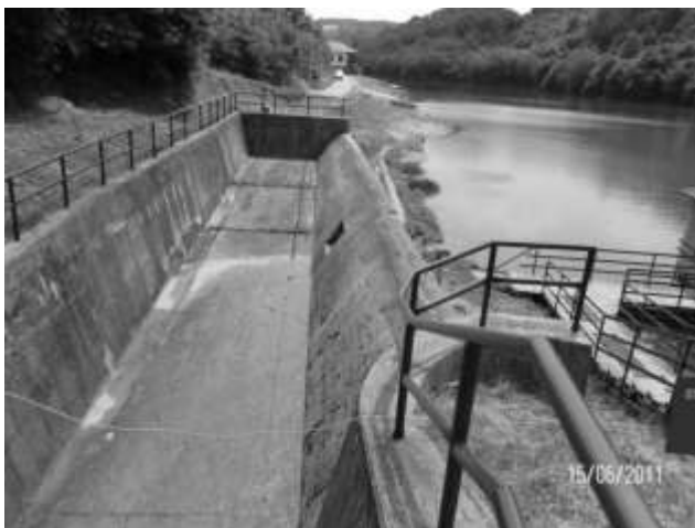
Figure 1. Emergency spillway; earthfill dam in the Barajevska Reka drainage basin (Photo: Đeković, 2011)
