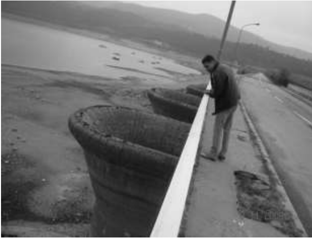
Figure 5. Frontal sinusoidal spillway, Dam Kokin Brod (Photo: Đeković, 2008)
