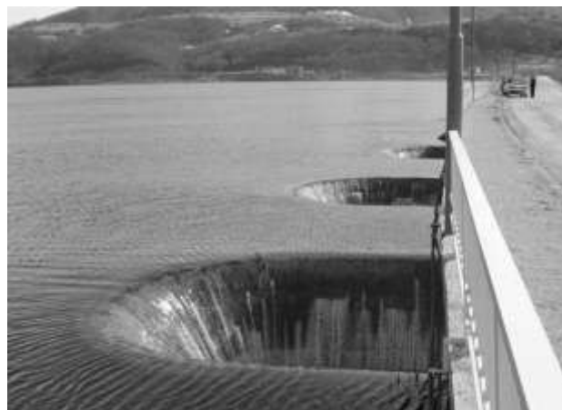
Figure 4. Spillway in the dam Kokin Brod; water level at the elevation of spillway crest (Photo: Đeković, 2010)
