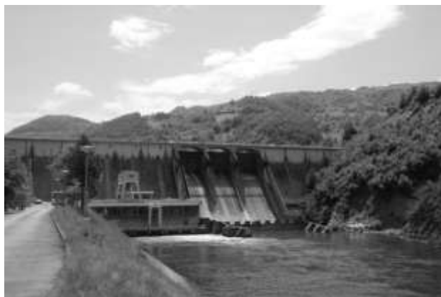
Figure 3. Segment gates in the spillway; Potpeć dam (Photo: Đeković, 2011)
